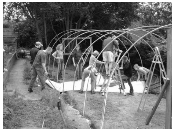
Trainees at Inishfree erecting a new polytunnel
